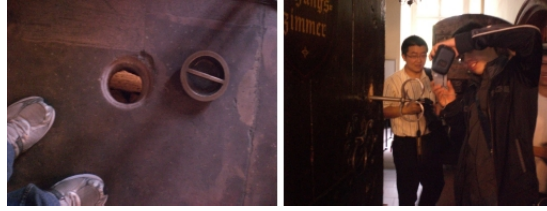
Figure 27: Left: The heating air will flow upward through the hole and warm the room. The round cover is beside the hole. Right: A huge key to a safe that secures the city's important documents.
